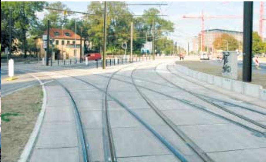
RSAG Rostock, Point covering Schröderplatz
