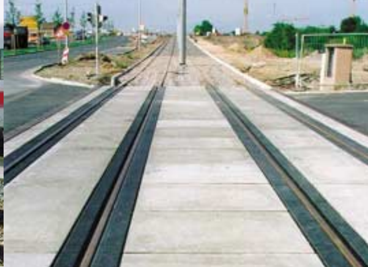
Rail crossing with elastomer edge section, Leipzig
