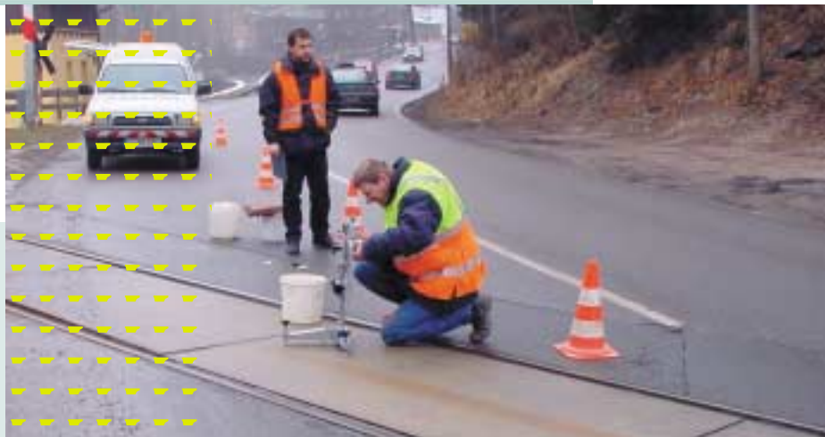
Measuring the SRT units
